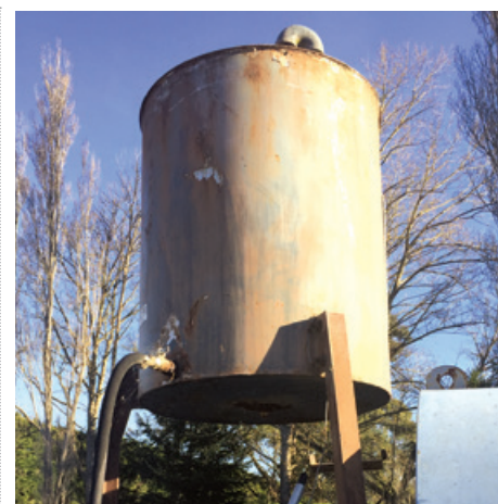
ABOVE: An example of a non compliant tank, which will have to be replaced
